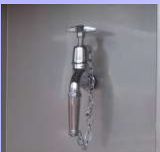
Chrome sampling tap fitted with in-line double check valve and insulated pipe-work pre-installed
